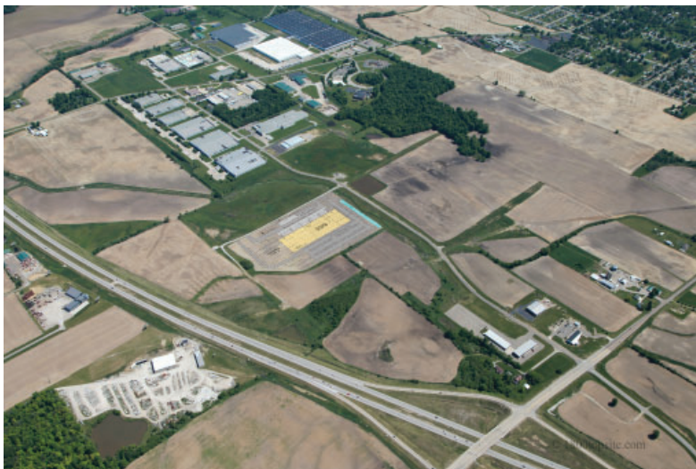
Magna Seating selected a SiteOhio authenticated site at Rock Mill Industrial Park in Lancaster, Ohio, for construction of its new automotive parts manufacturing facility, which will employ 300 workers.
