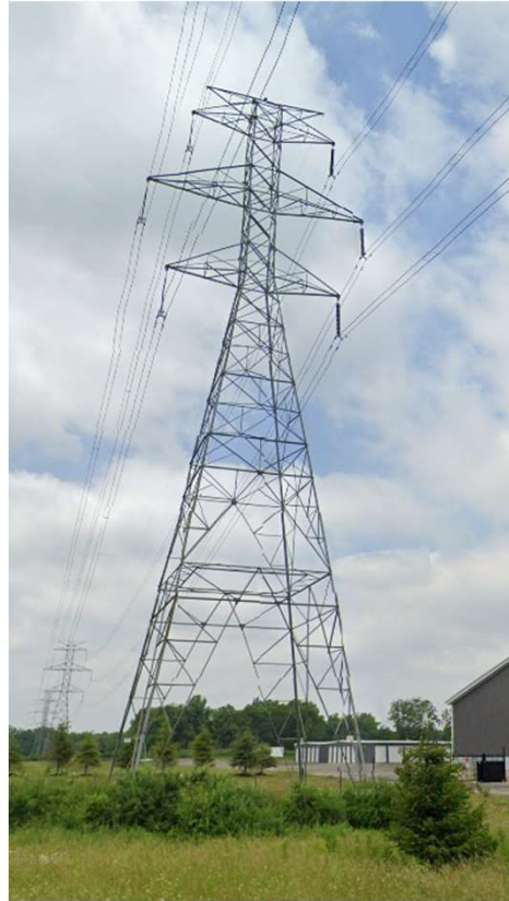
345kV Double-Circuit Steel Lattice Structure with 2-Bundle Conductor
