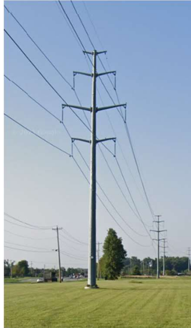
138kV Double-Circuit Monopole Structure
