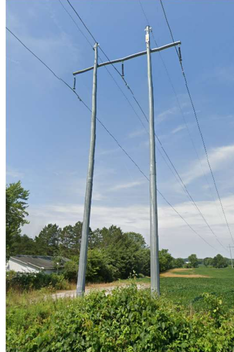
138kV Single-Circuit H-Frame Structure
