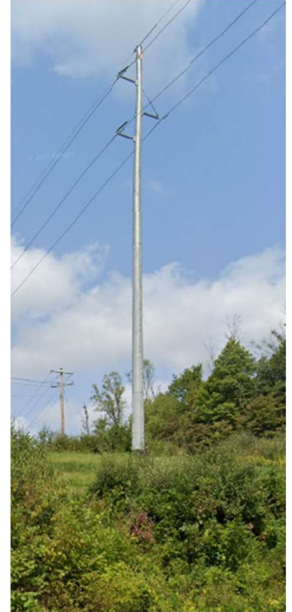
138kV Single-Circuit Monopole Structure
