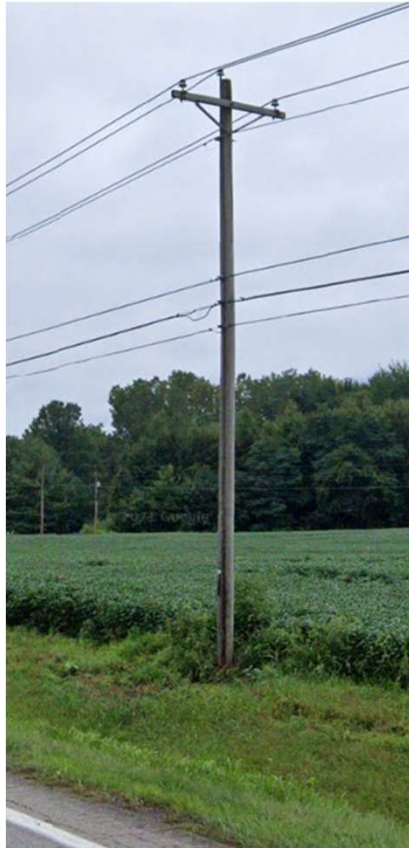
12kV Single-Circuit Three-Phase Distribution Line
