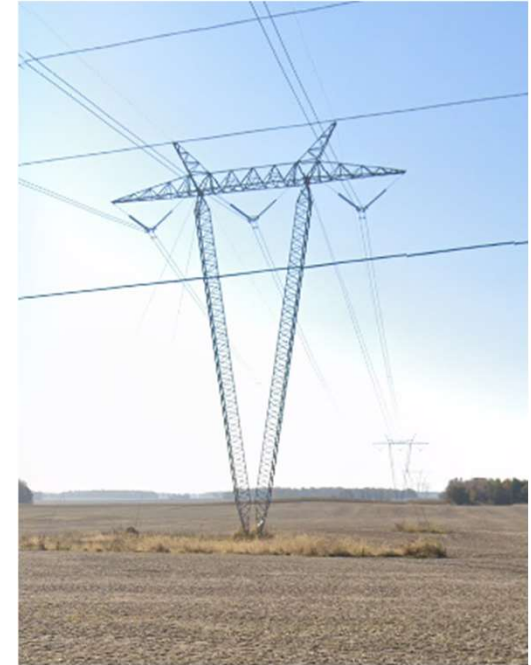
345kV Single-Circuit Guyed-V Structure with 2-Bundle Conductor
