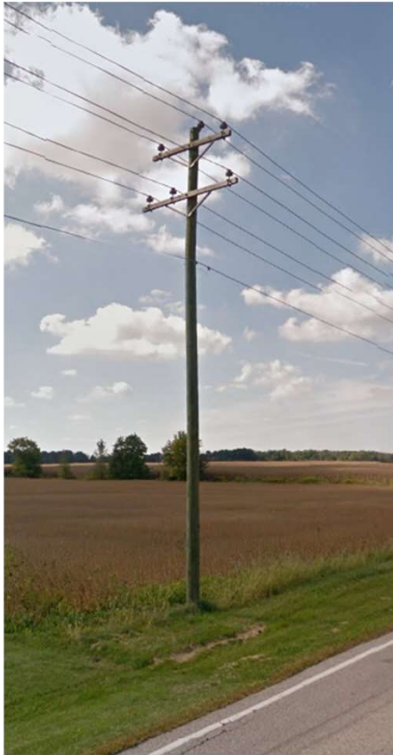
25kV Double-Circuit Three-Phase Distribution Line
