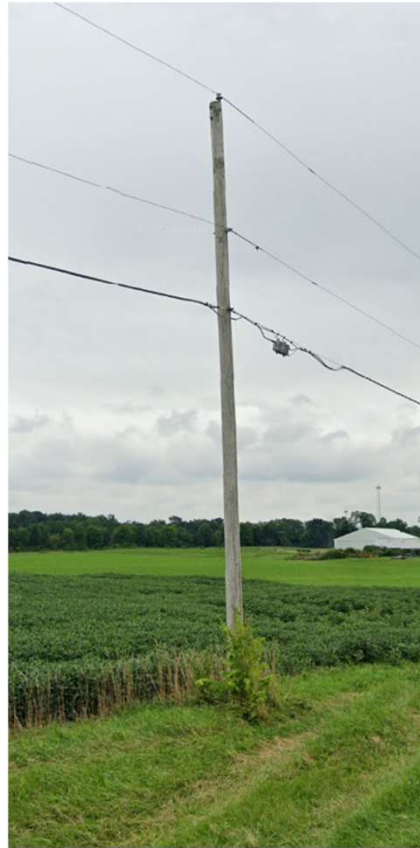
7.2kV Single-Phase Distribution Line
