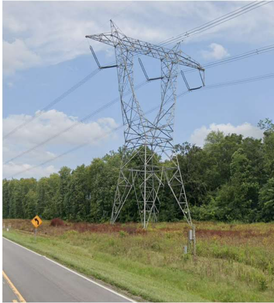
765kV Single-Circuit Steel Lattice Structure with 4-Bundle Conductor
