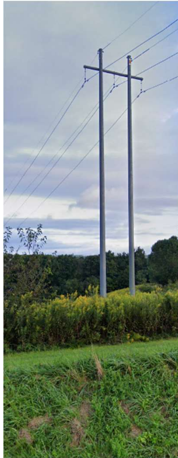
69kV Single-Circuit H-Frame Structure
